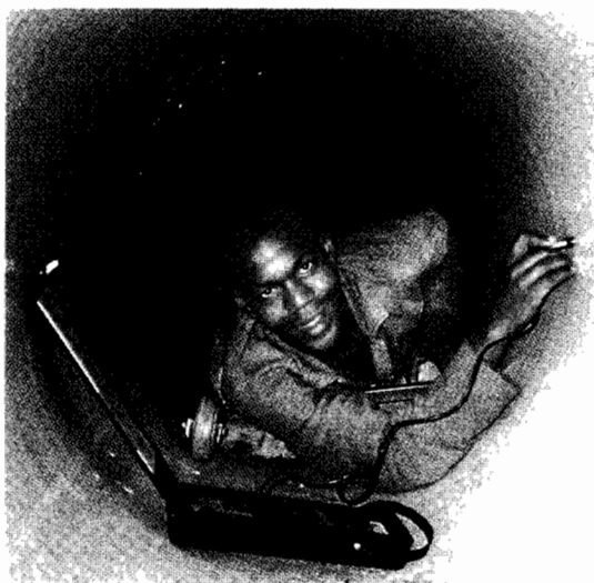
Epoxy applied after removal of the failed bitumen lining
